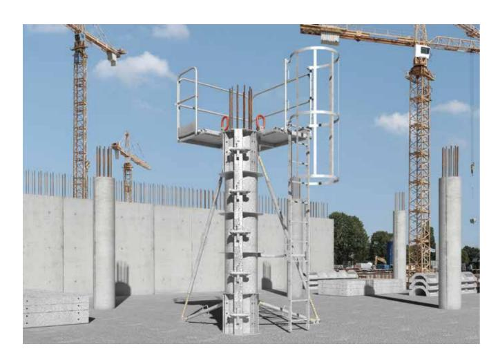
The implementation of circular formworking from standard galvanised steel components is straightforward with Pilco® columns formworking.
